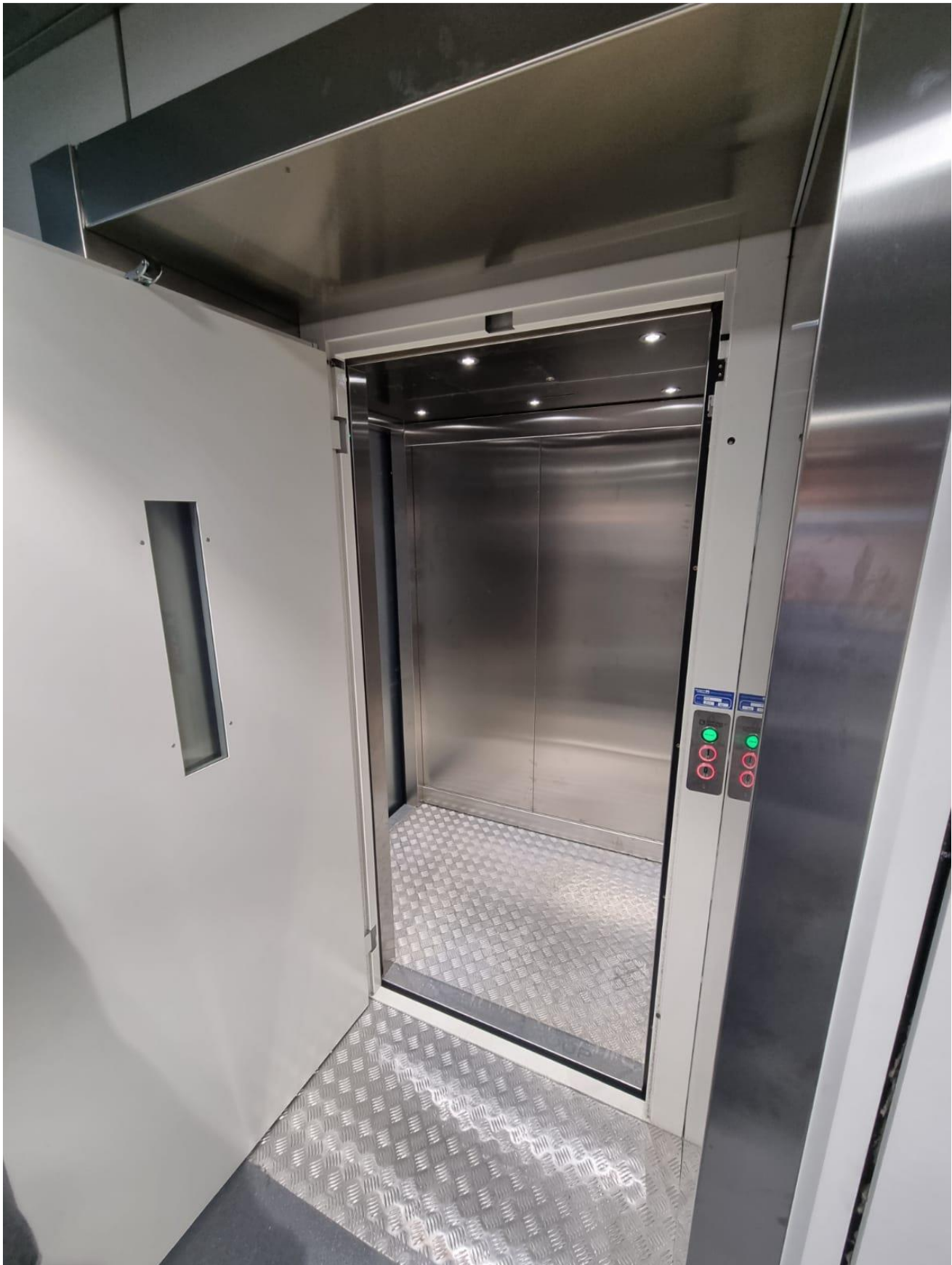
Image 3. Freight elevator, pier level
