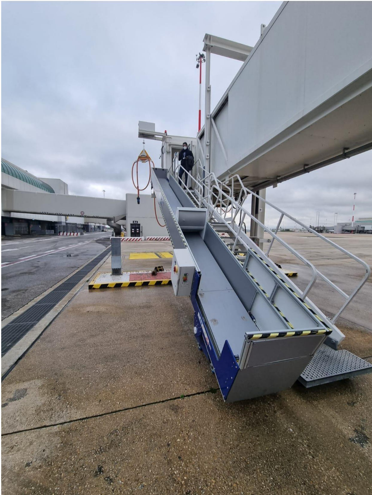
Image 1. Motorised slide installed at a landing stage, runway level
