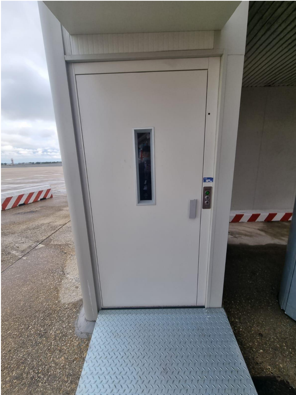
Image 2. Goods lift, runway level
