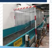
On the section of the baggage claim belt prior to baggage unloading on the carousel where it is picked up by passengers, an automatic device has been installed to dispense a hypochloric acid-based sanitizing mist based that is released when baggage passes through a tunnel.
